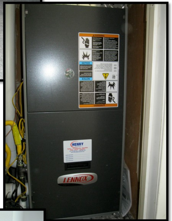
Fig. 3— Replaced old gas furnace with a new 95% energy efficient furnace with a smart thermostat. (above).
