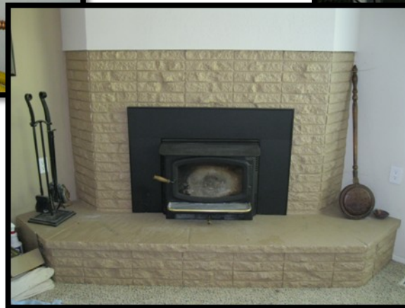
Fig. 4— Replaced old wood stove with new high biomass wood stove taking him from 2.5 to 1.5 cords (above)
