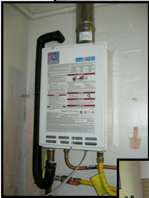
Fig. 2— Replaced old gas heater with on-demand energy efficient model. (above)
