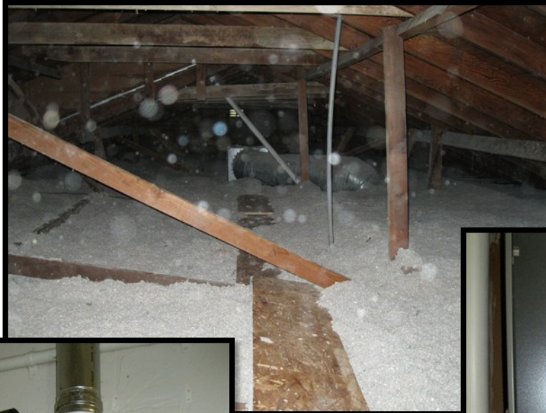
Fig. 1—12” blown insulation added to attic (left)
