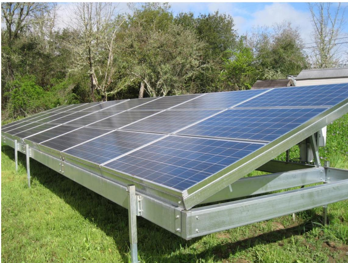
**The Solution:** Once the Sun-Pods had been delivered and set on the ground, Synergy began the installation. The Sun-Pods come with the racking and panels factory installed and ready. Synergy first installed the SMA inverter that has the mounting brackets on the Sun-Pod but is installed in the field. The footing legs were tacked down with 18” Galvanized rebar to secure the Sun-Pods to the ground.
